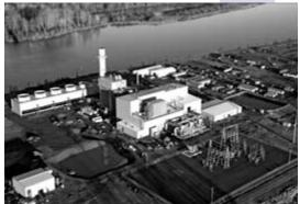
Port Westward, our new 400-megawatt natural gas-fired plant, has a G-class turbine, making it the most efficient natural gas plant in the Pacific Northwest.
